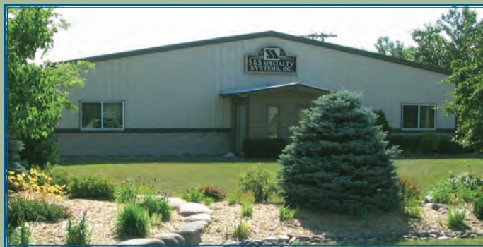
The S&S Specialty Systems manufacturing plant in Iron River, WI.
